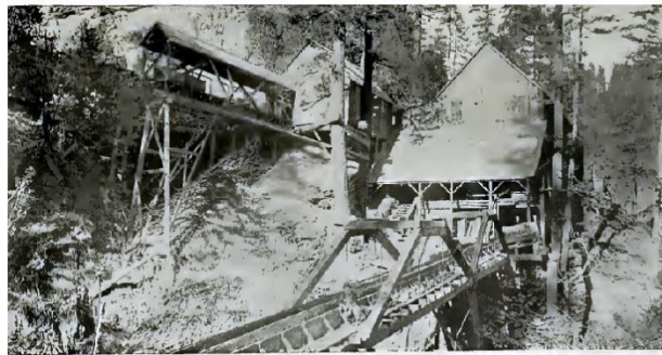
GRAVEL WASHING PLANT, HIDDEN TREASURE MINE, PLACER COUNTY, CAL.
