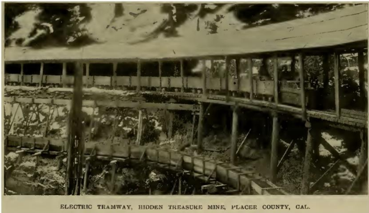
ELECTRIC TRAMWAY, HIDDEN TREASURE MINE, PLACER COUNTY, CAL.
